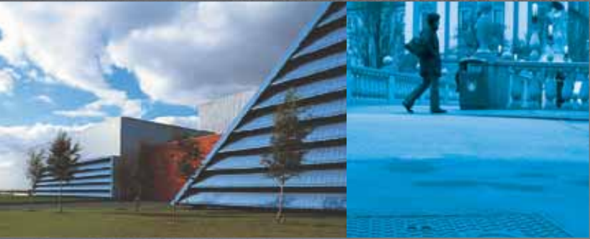
TELECOM & CABLE NETWORKS
